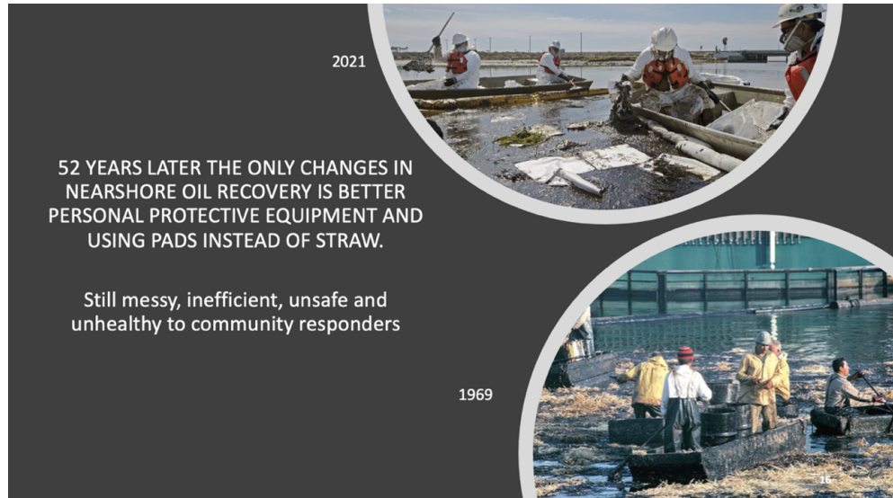
Figure 2 - Shore zone recovery of mobile crude oil: rakes, shovels, sorbents and open storage containers 1969 Santa Barbara Oil-rig Blowout, 2021 Orange County Pipeline Spill
